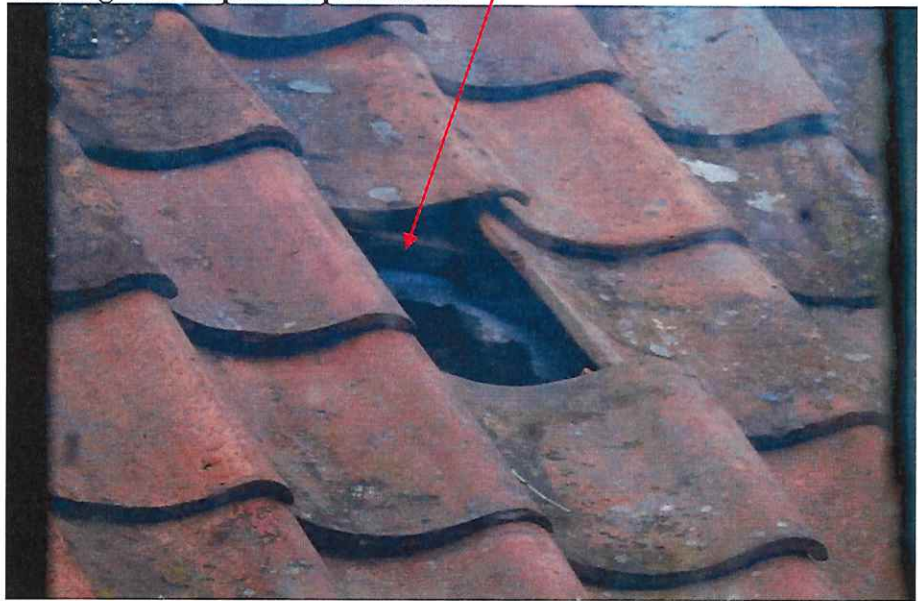
Missing tiles require replacement
