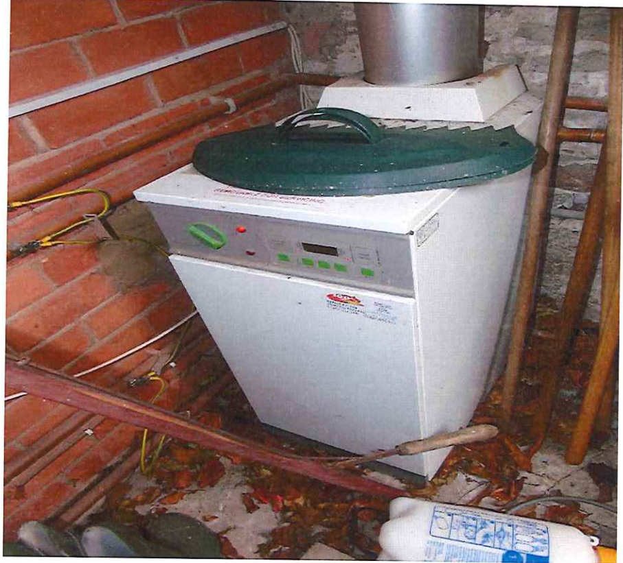
Oil fired boiler in store shed
