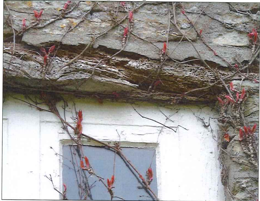
Severely infested lintel – top floor right hand flank wall
