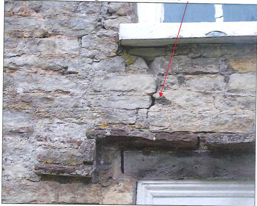
Cracks/distortion over ground floor windows
