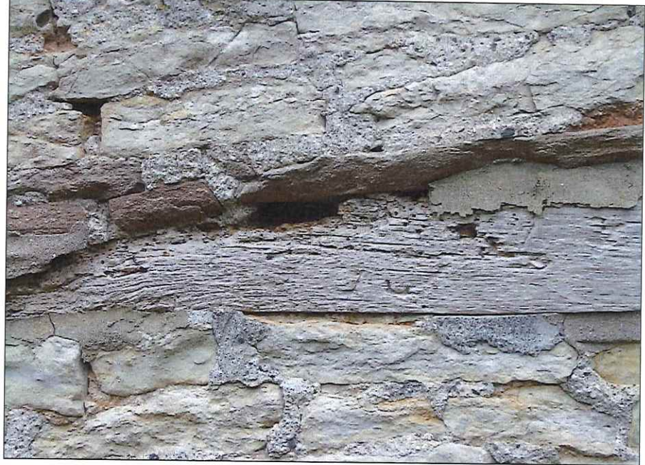
Severely infested lintel – top floor right hand flank wall
