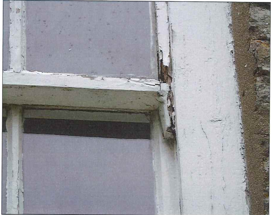
Rotten joinery – left hand windows
