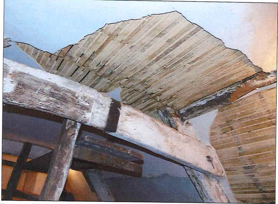
Poor ceiling – rear attic room
