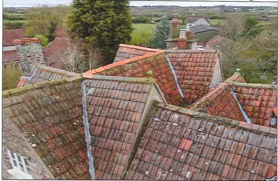
Aerial Photograph General view of roof – note distorted ridges
