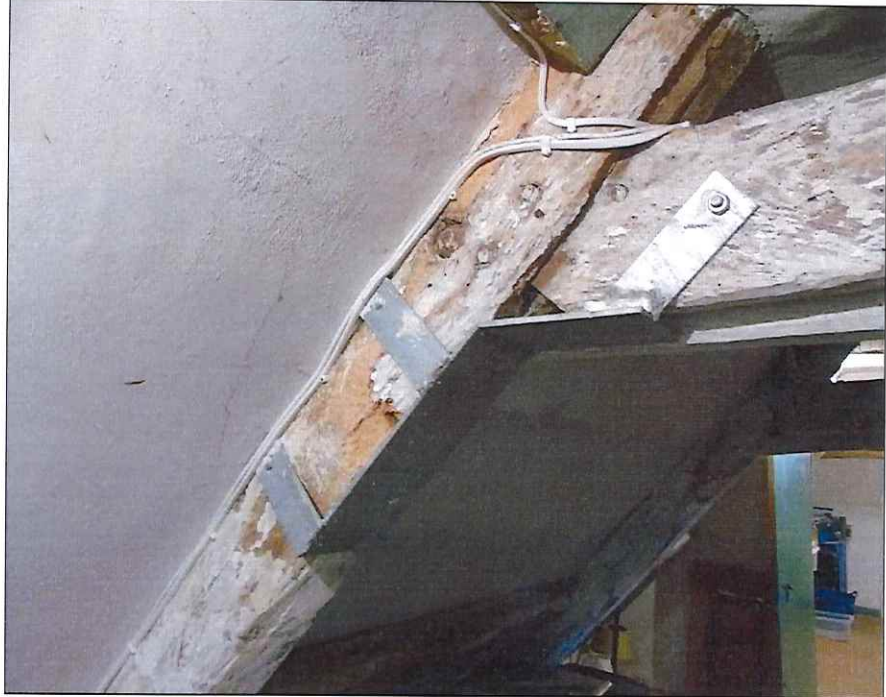
Bracing on roof timbres
