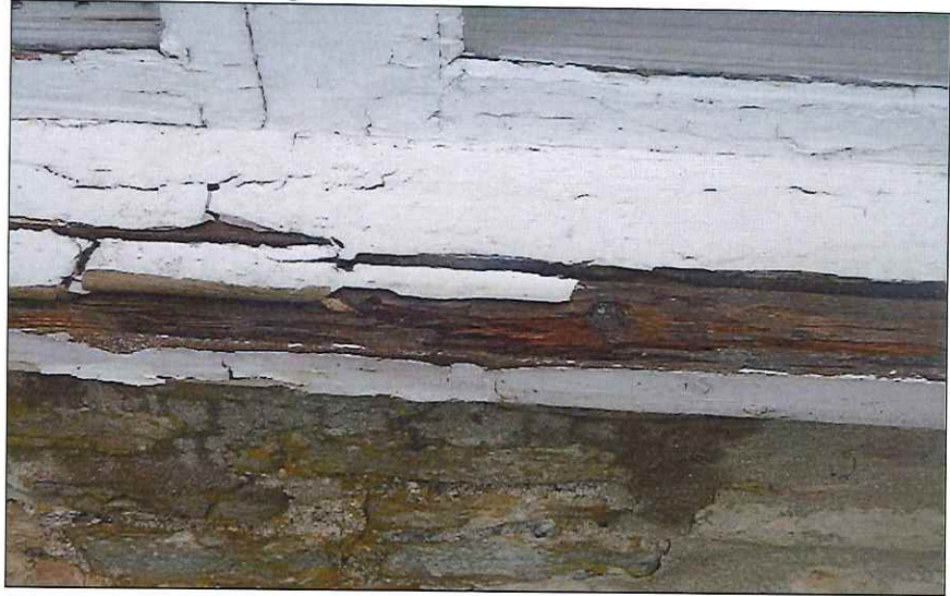
Rotten joinery – left hand windows
