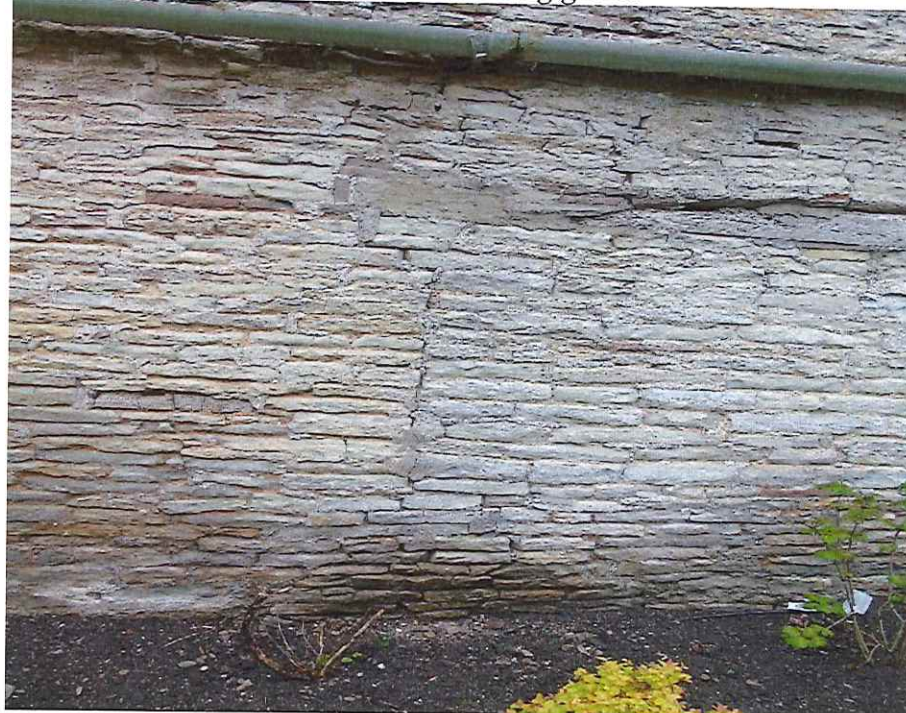
Stains on lower rear wall due to leaking gutter
