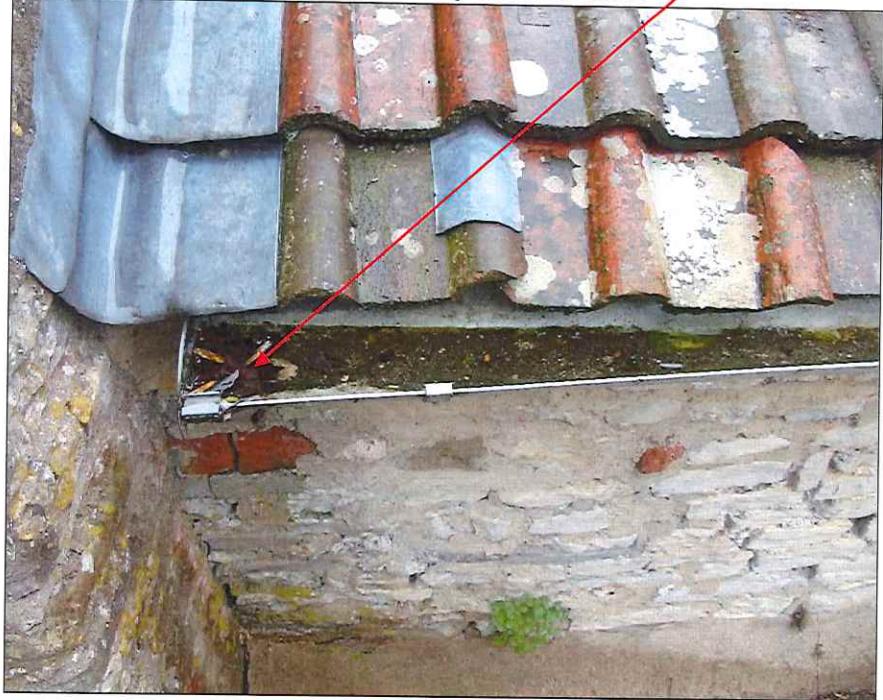
Uneven gutter – rear single storey kitchen roof
