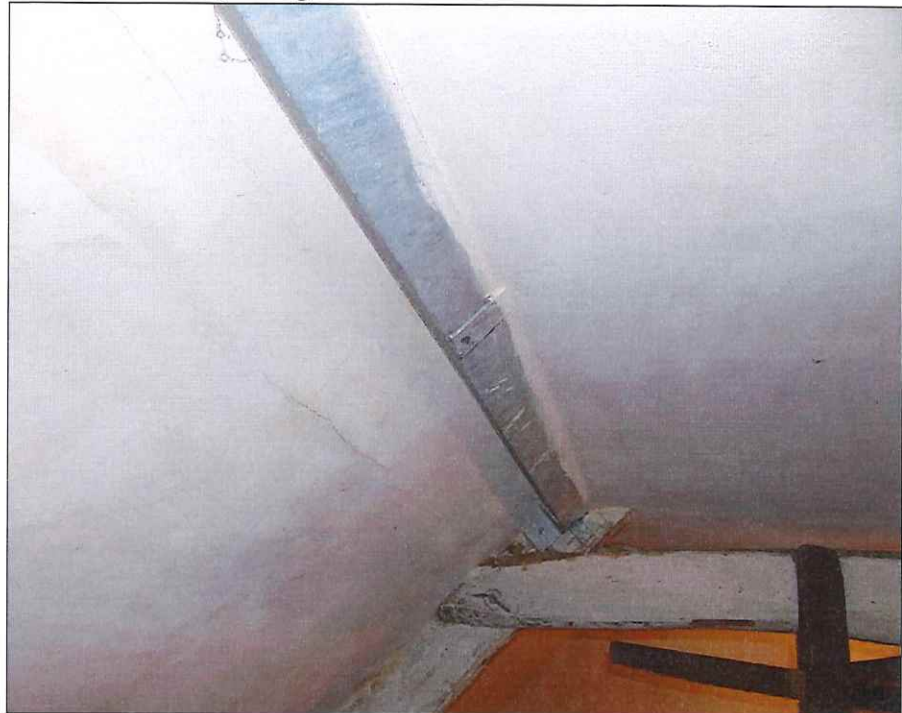
Modern bracing in right hand loft room
