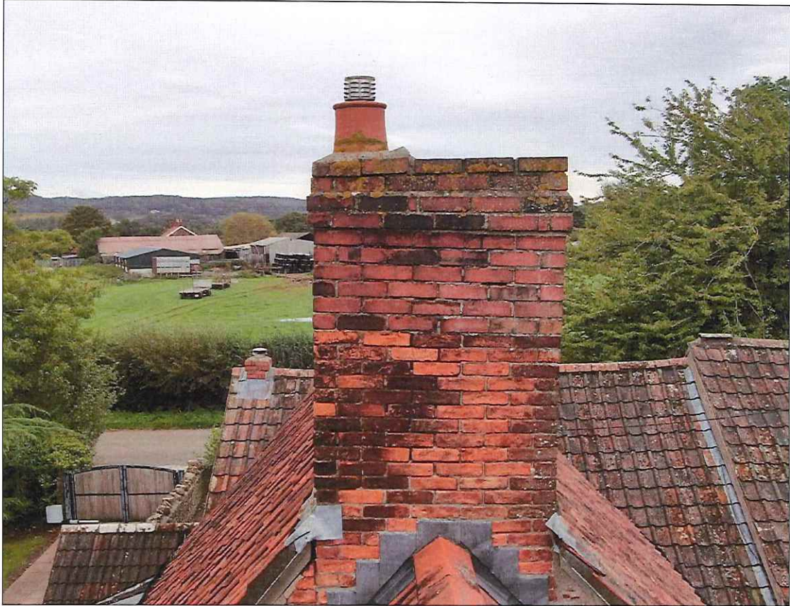
Large front right hand stack – open flue and poor pointing
