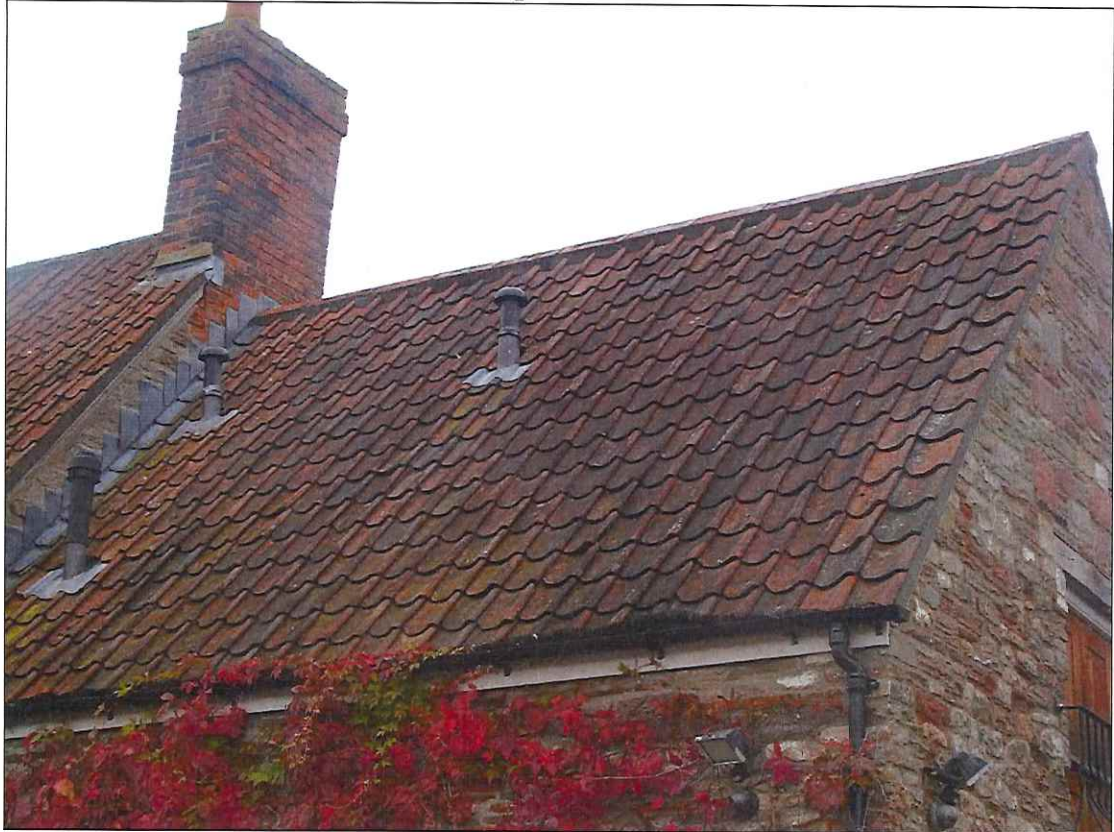
Roof of rear “annex” – right hand slope
