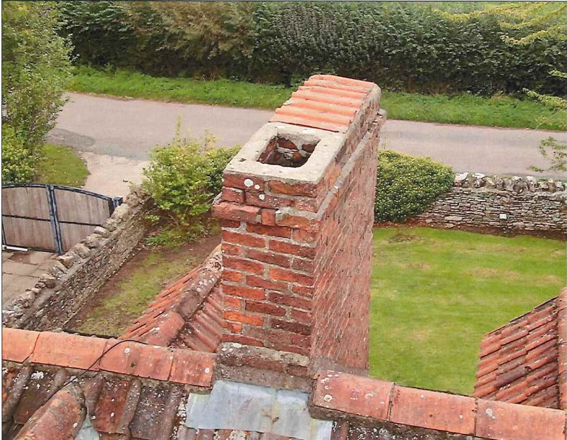
Large front right hand stack – open flue and poor pointing
