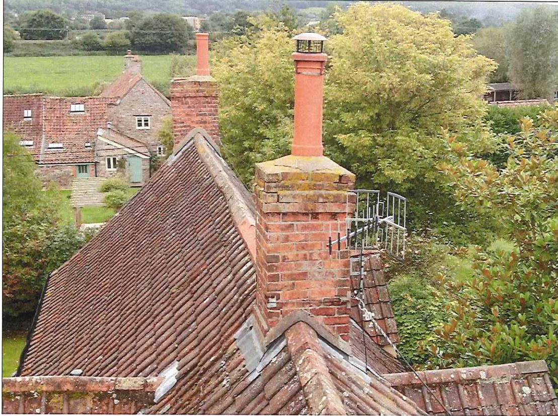
View of roof/chimney looking west
