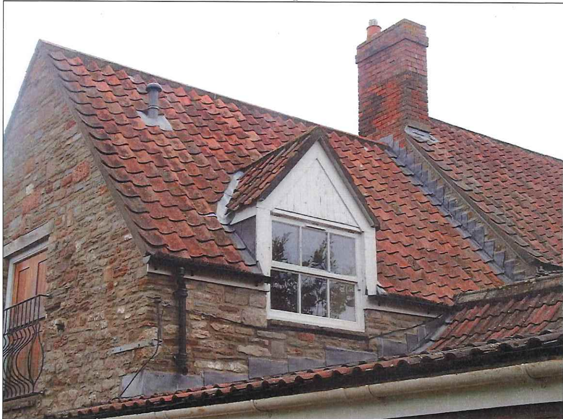
Roof/dormer of rear “annex” left hand slope
