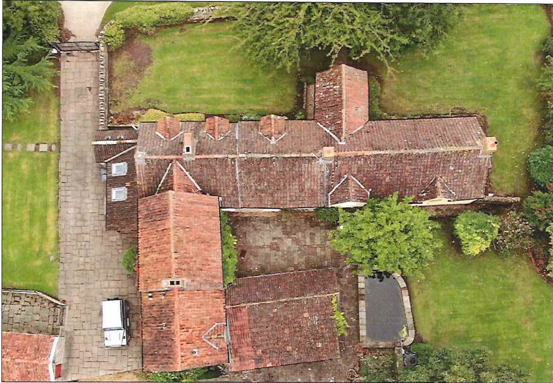
Aerial view of roof
