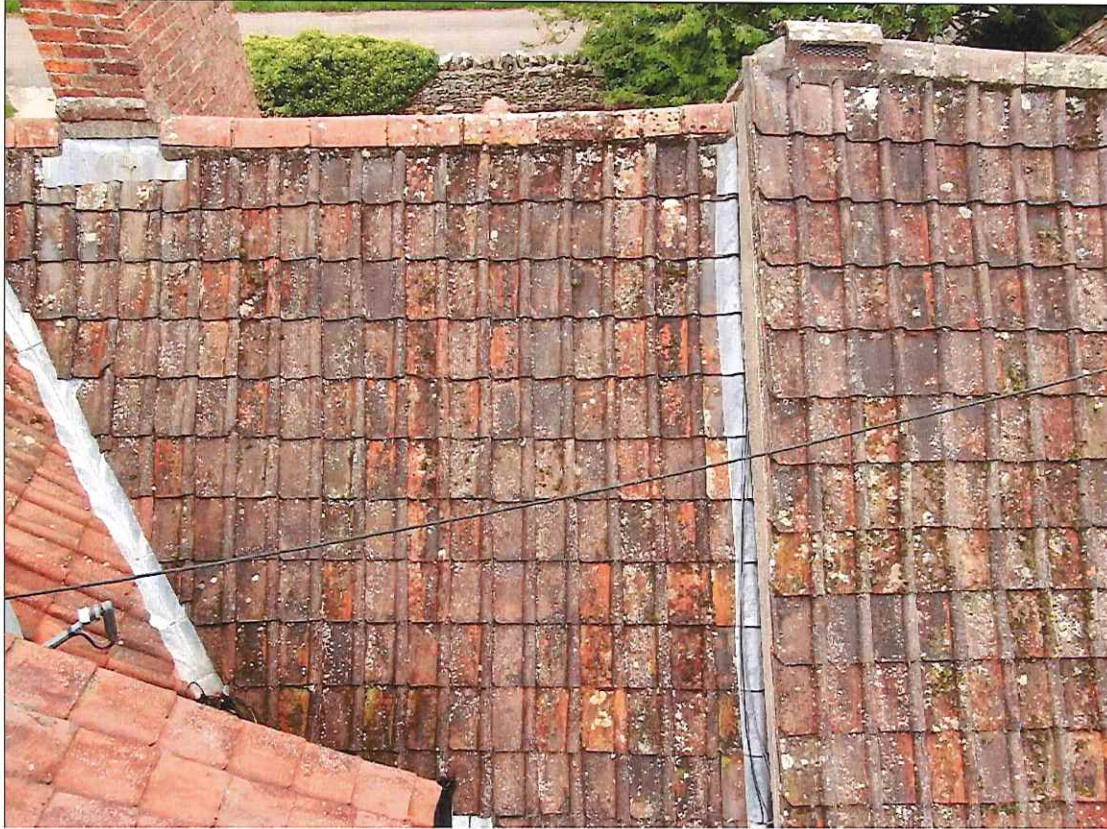
Rear roof slope – general view
