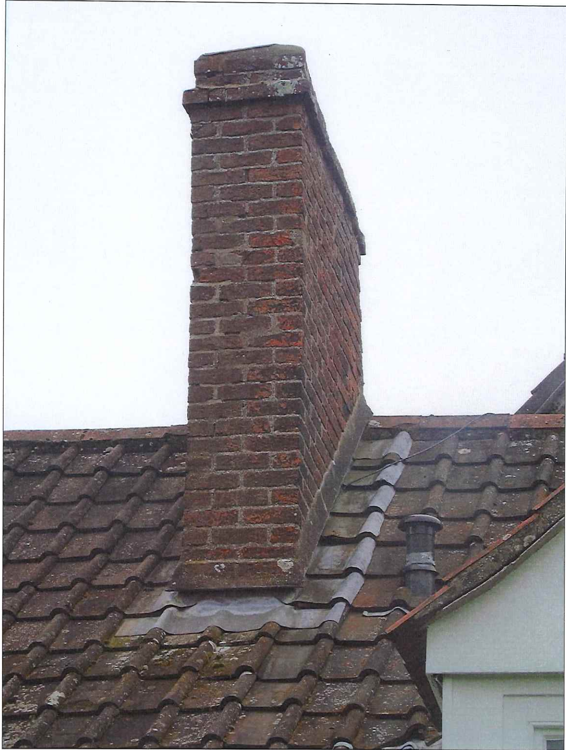
Front right hand (large) stack
