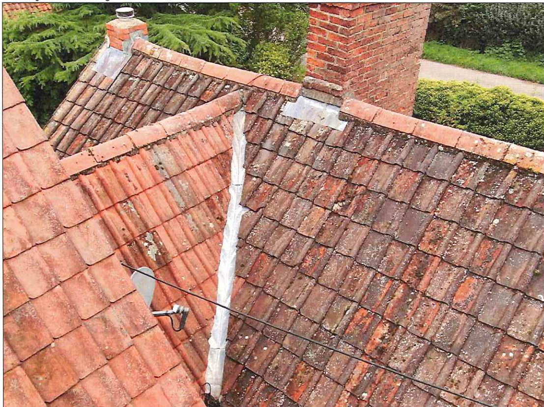
Valley detail at joint between main roof and “annex”
