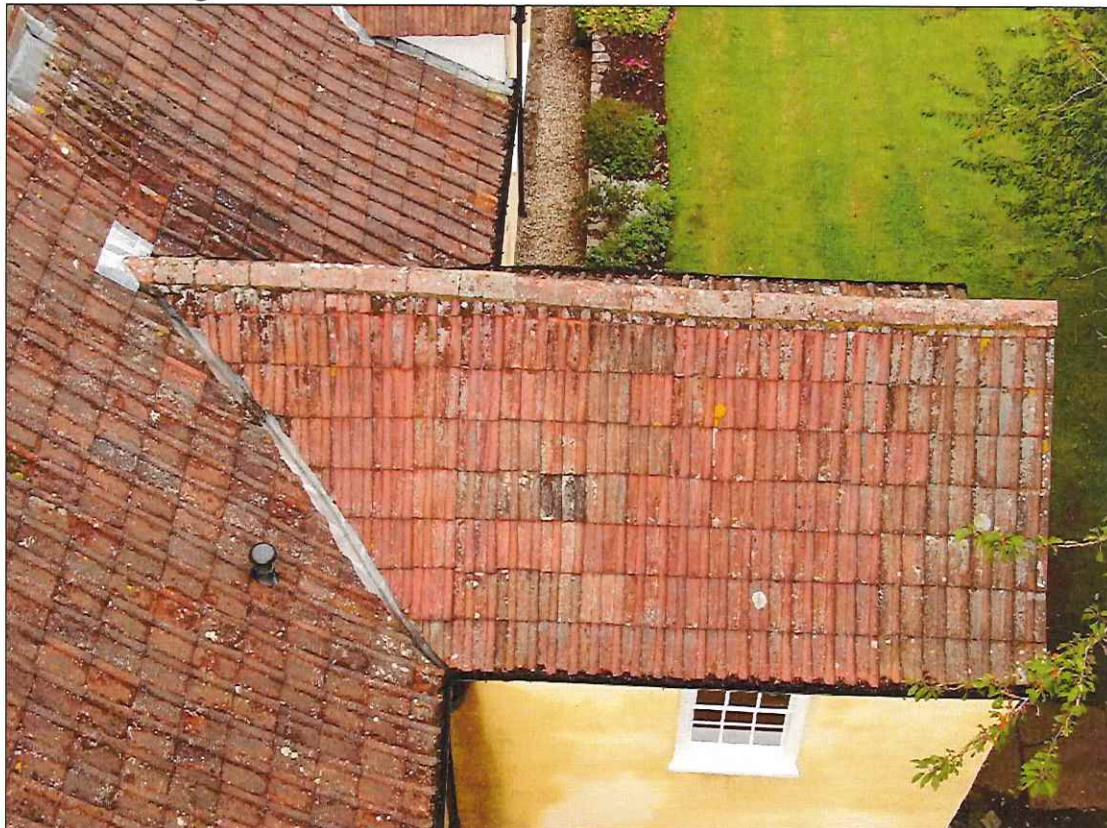
View of front gable roof
